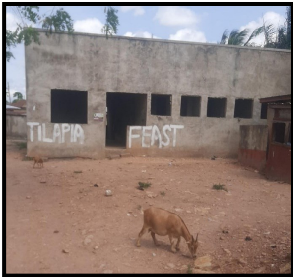
Plate 2: Construction of a new toilet facility close to Kpong Wharf is on hold due to legal issues.
