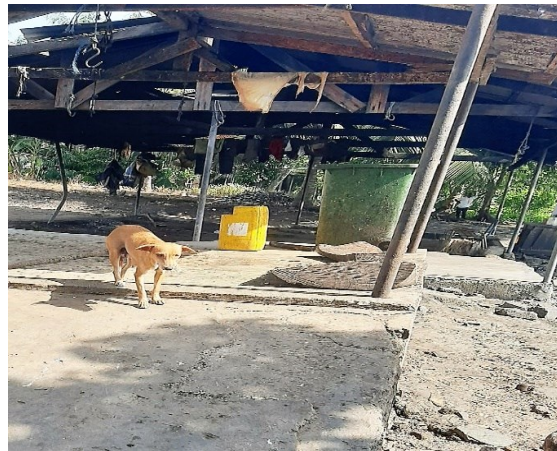
Stray animals have access to exposed slaughterhouse shed at Atimpoku
