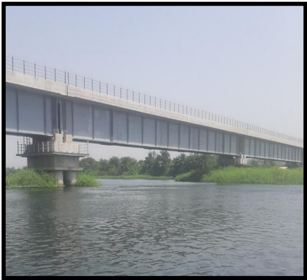
Plate 4: Newly constructed Bridge at Senchi has begun trapping aquatic weeds.
